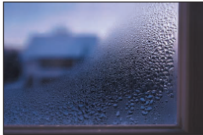
Condensation on the inside of a window-pane.
