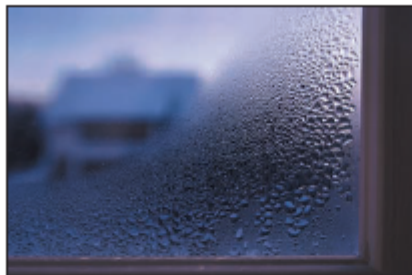
Condensation on the inside of a window-pane.
