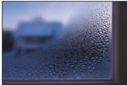
Condensation on the inside of a window-pane.
